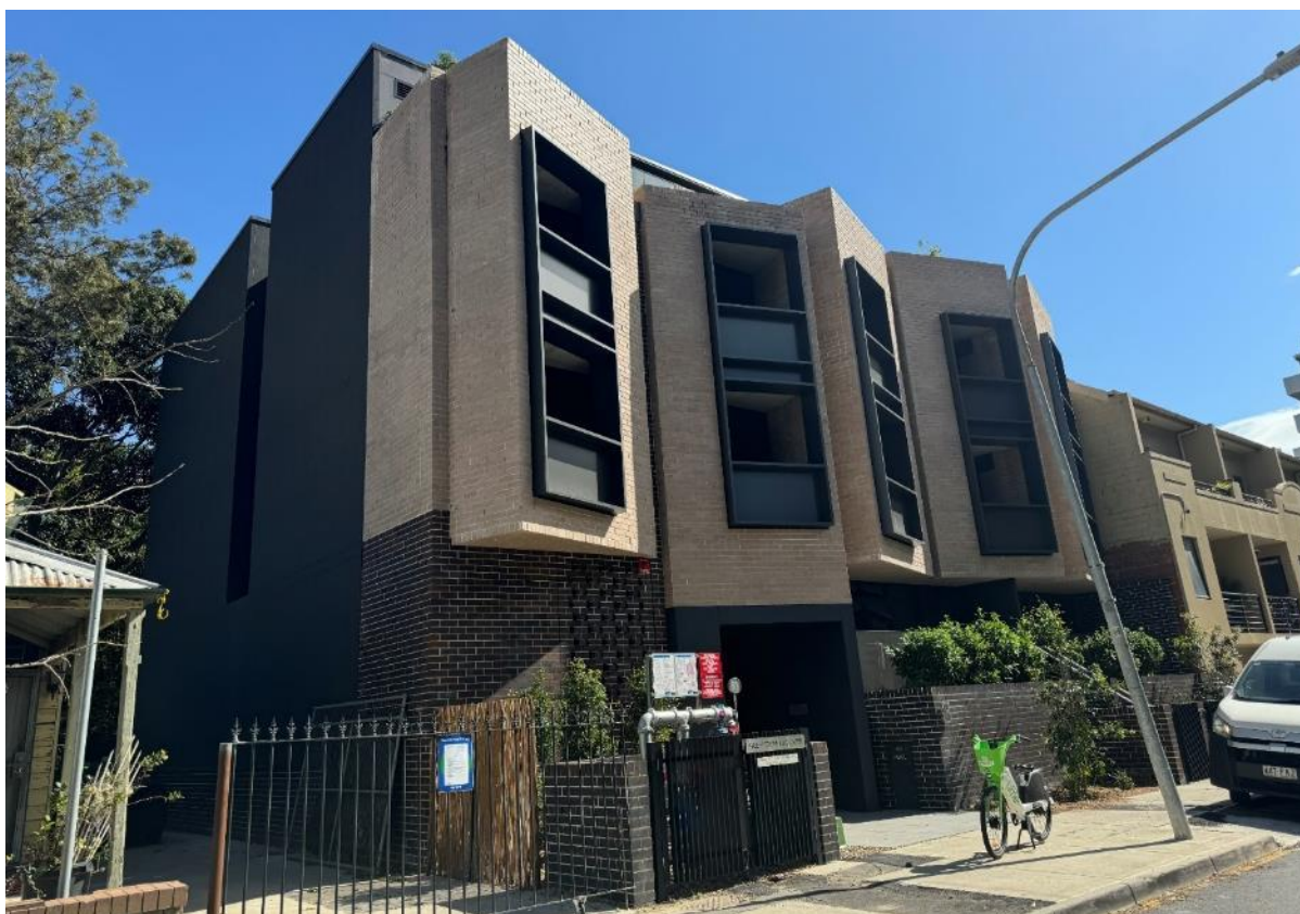
Figure 7: Neighbouring property at 1-3 Goddard Street
