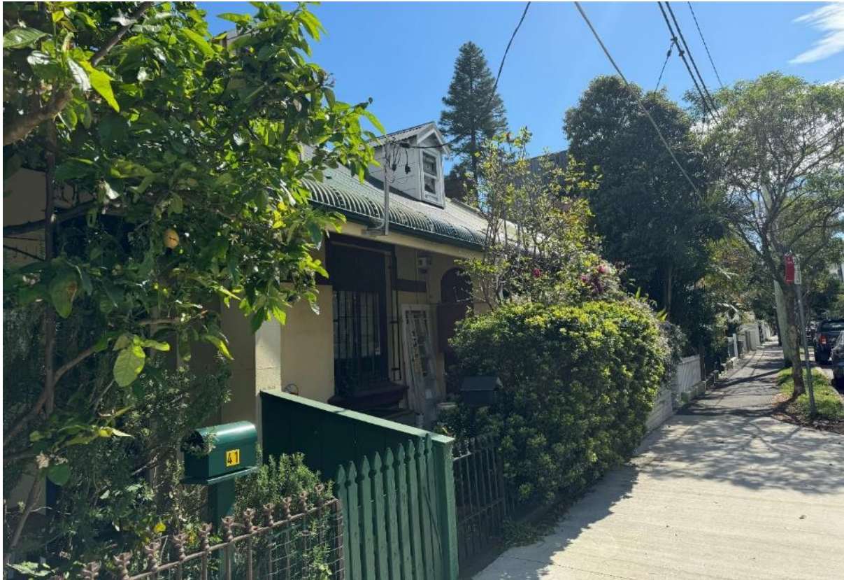
Figure 13: Neighbouring properties at 27-41 Eve Street
