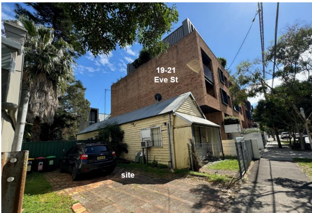
Figure 4: Site (23 Eve Street) viewed from Eve Street, and 19-21 Eve Street in the background
