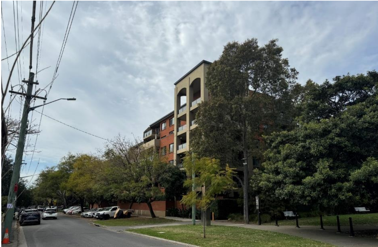
Figure 11: Neighbouring property at 177-219 Mitchell Road
