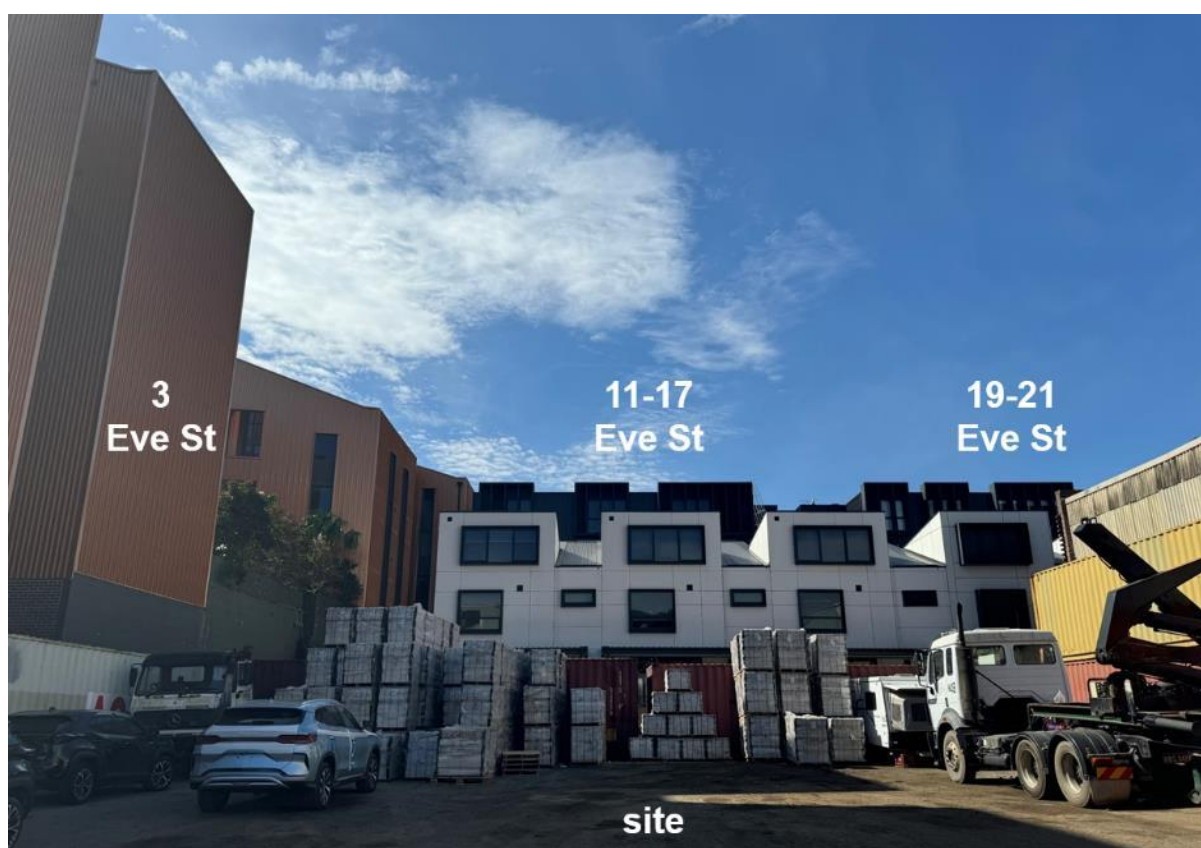
Figure 8: Neighbouring properties at 3, 11-17 and 19-21 Eve Street, viewed from the site (internally)
